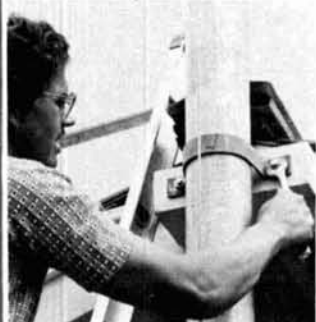
Mounting the House Bracket
